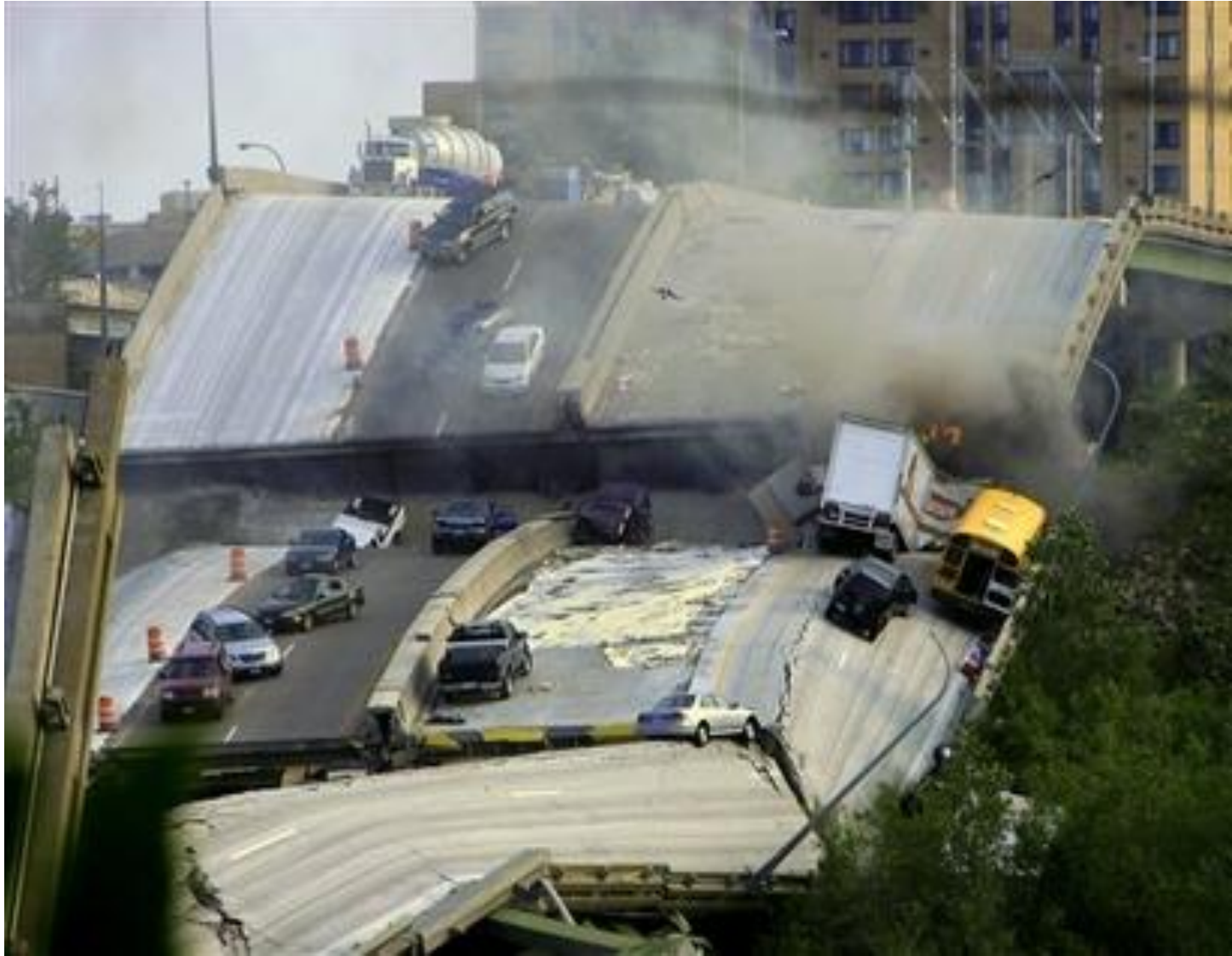
Minneapolis bridge collapse, Aug 1, 2007 3
